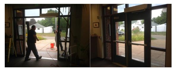
The entrance doors to Central Office were replaced and a safety buzzer system installed. This entrance was the last entrance on the school campus to have a buzzer entrance installed as a security measure. Replacing the rusted doors also will add to the energy efficiency this winter.
