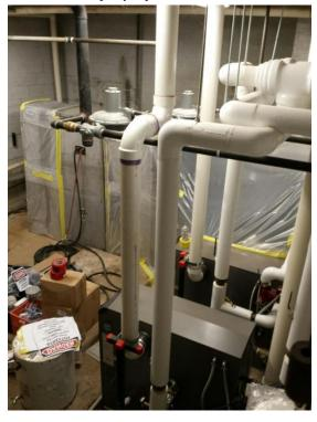
Although never seen nor visited, this space needed to be made asbestos free. The team moved in with air scrubbing units, plastic protection barriers and all the equipment necessary to remove the asbestos wrappings from the subterranean pipes.
